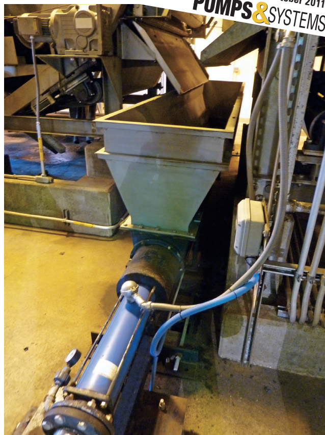
The progressive cavity cake pump with a reinforced hopper
